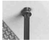
Stainless steel screws draw door frame tight.
